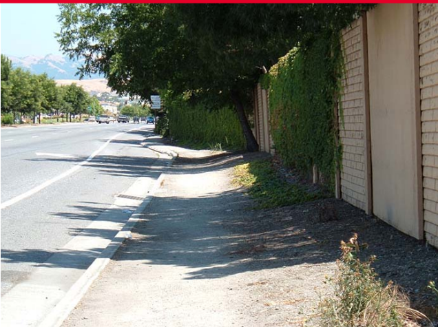
Looking east from Narvaez Avenue toward Bluefield Drive
