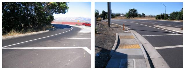
**Photos:** Unsafe intersection redesign forces people to walk in the traffic lane of a blind turn (left photo, NW corner) or the fast right-turn lane (right photo, SW corner). [more photos]
